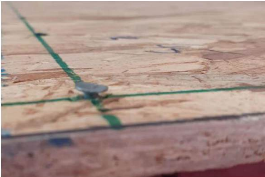
Figure 4. Lifted nail heads.
